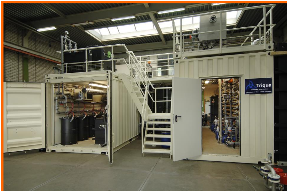
Overview Sewage Treatment Plant
