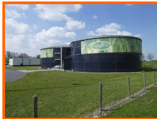
Bioreactor and buffertank FrieslandCampina Maasdam
