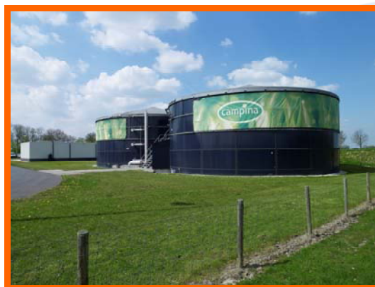
Bioreactor and buffertank FrieslandCampina Maasdam
